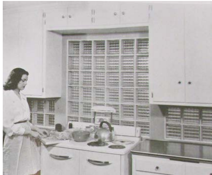
Figures 87 & 88 - Above: Use of glass block as an infill material, Below: Use of glass block in the kitchen, 1945 (from “Beautiful Homes”, trade catalog by Owens-Illinois, published 1945)
