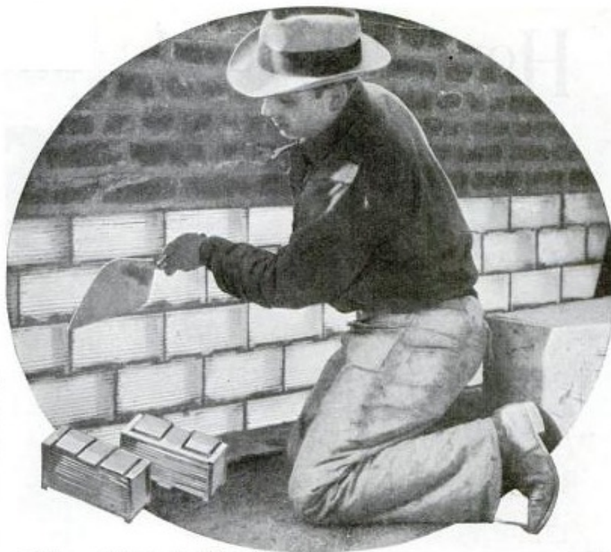
Figure 14 - Installation of glass blocks at the roof of the Barbizon Plaza Hotel (published in "Glass Walls Now Used in Building", Popular Science , June, 1930)
