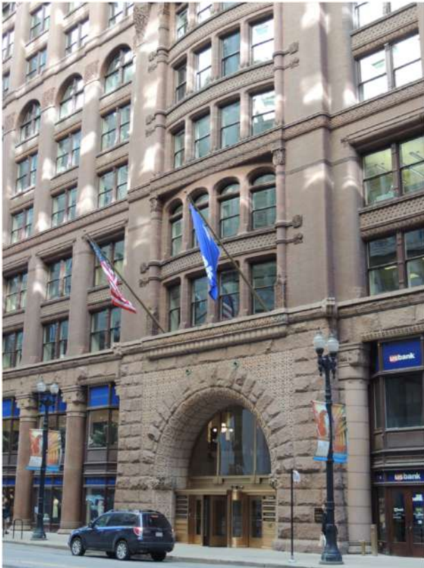
LaSalle Street Entrance; photo by Jean Follett
